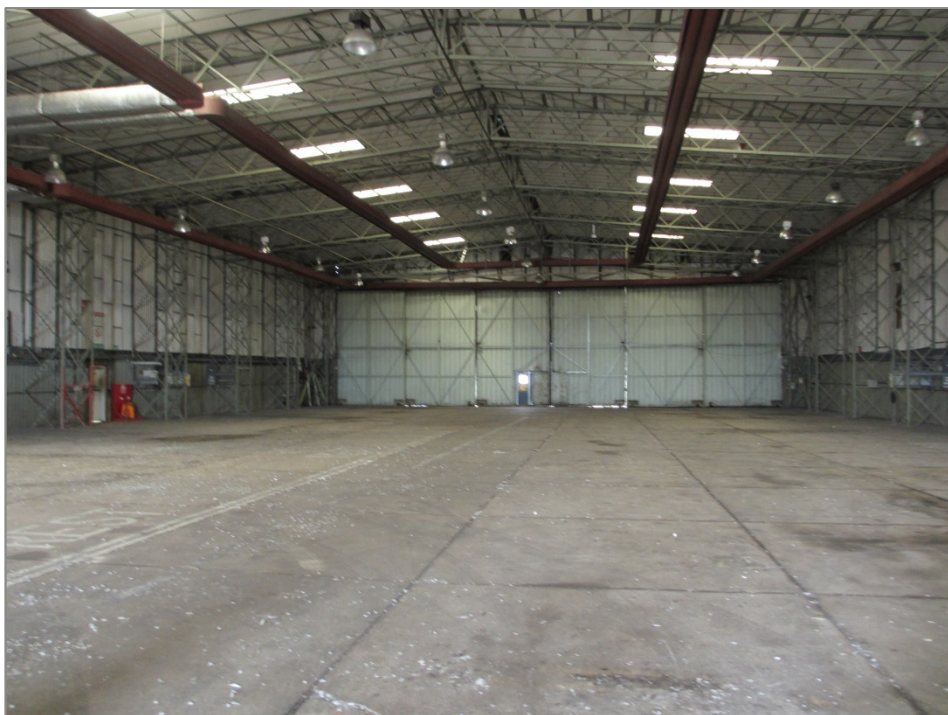
Figure 18: First cargo hangar interior
