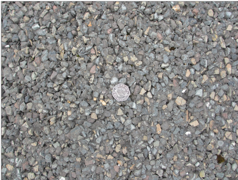
Figure: 9 Large aggregate used for wearing course may be impacting surface friction characteristics
